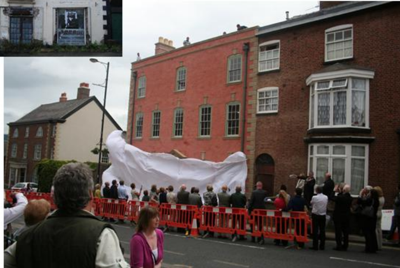
Mostyn House, Vale Street, Denbigh, a Grade II fine town house – historical research and uncovering of features during works returned the character of the building back to its Georgian origins
